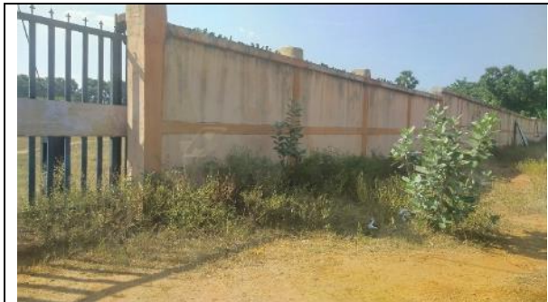
Figure 5-3- Green Hydrogen Hub Site – Main Gate
